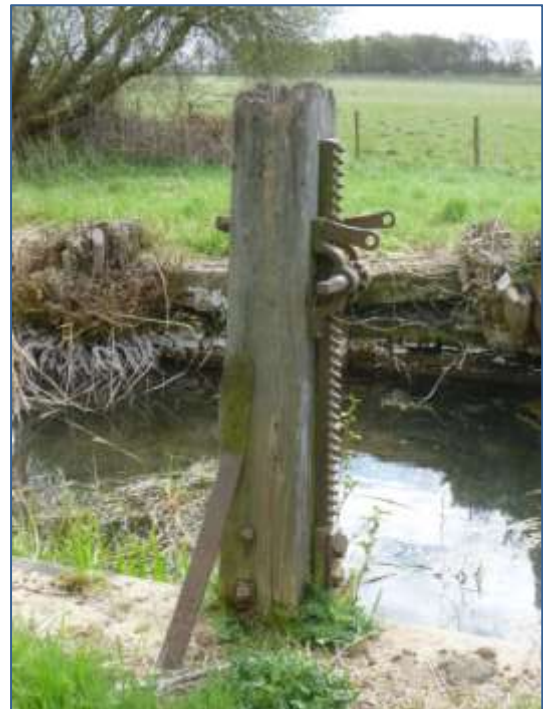
Plates 38-39: Ground paddle gear at Top Lock (left) and Sandhill Lock (right)
