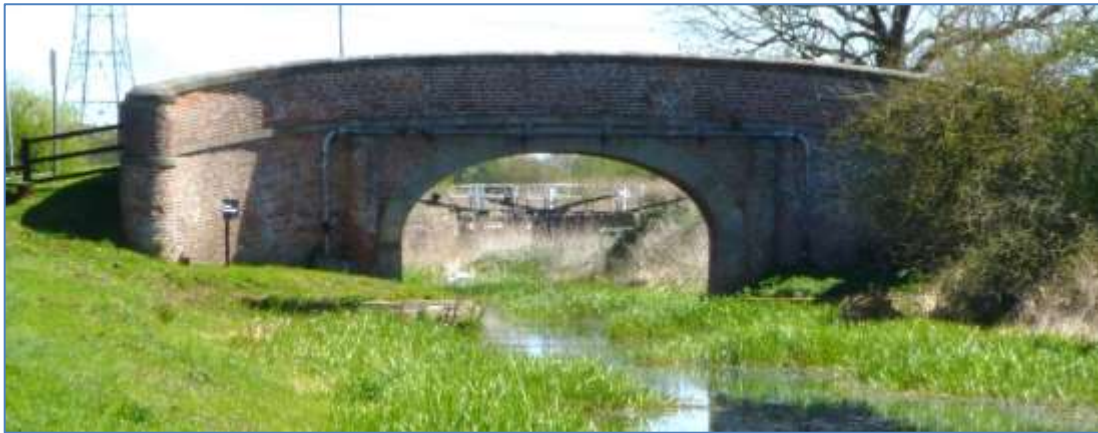
Church Bridge (HA22) and Thornton Lock (HA19)
