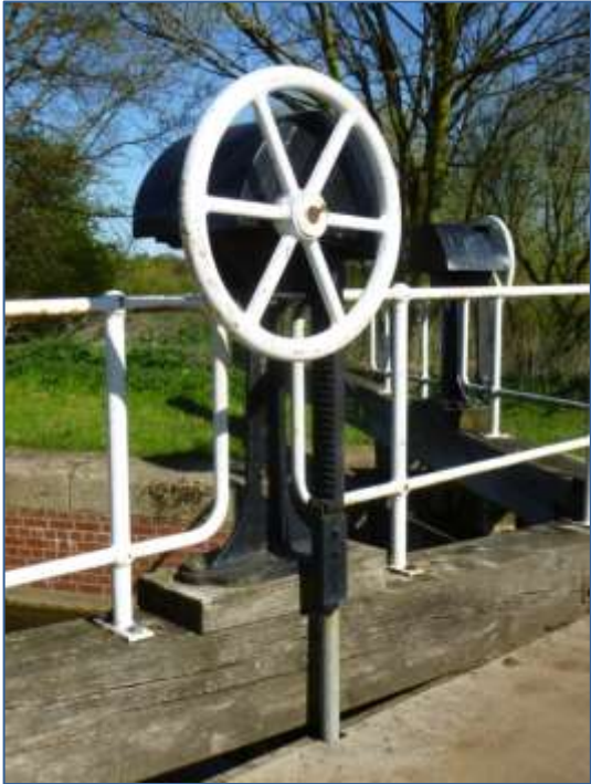
Plates 40-41: Gate paddle gear at Cottingwith Lock (left) and Gardham Lock (right).
