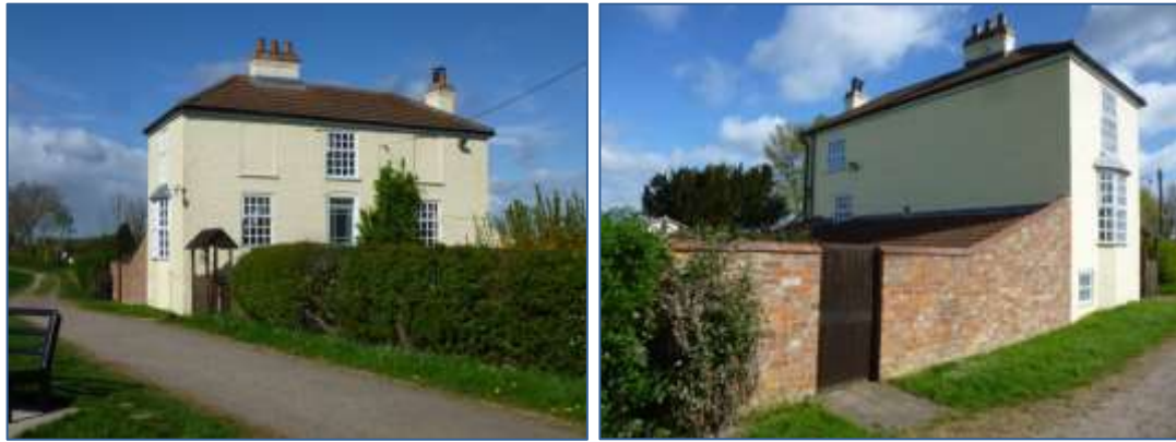
Plates 47-48: Lock Keepers Cottage (HA 3)
