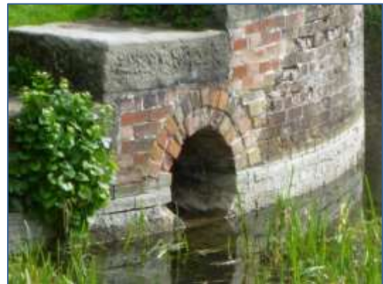
Plates 36-37: Example of square profile (left) and circular (right) outfalls from by-washes at Walbut Lock and Silburn Lock.
