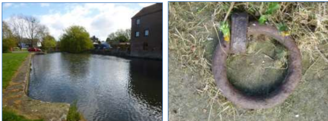
Plates 16-17: Canal Head (left) and detail of ring cleat (right)
