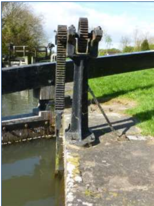
Plates 38-39: Ground paddle gear at Top Lock (left) and Sandhill Lock (right)
