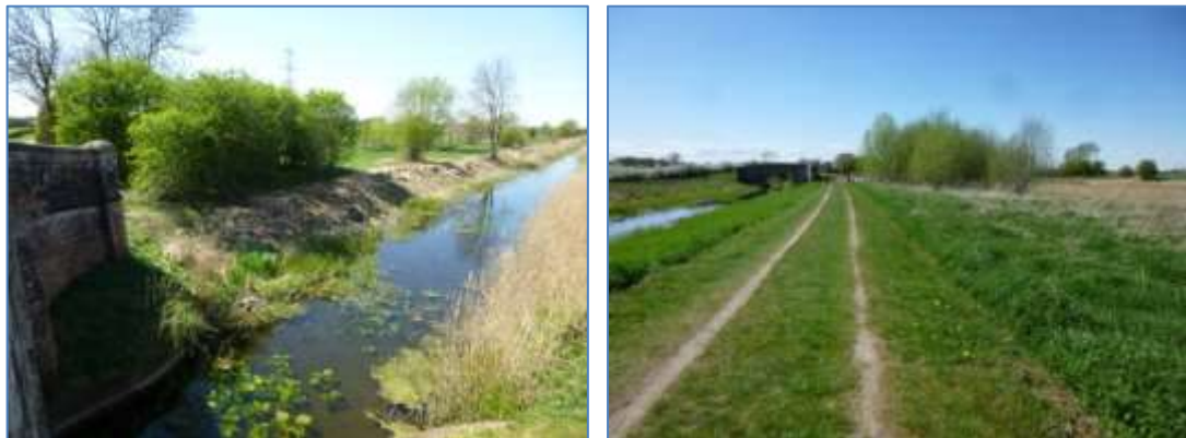
Plates 22-23: Minor wharfs at Walbut Bridge (left) and Church Bridge (right)
