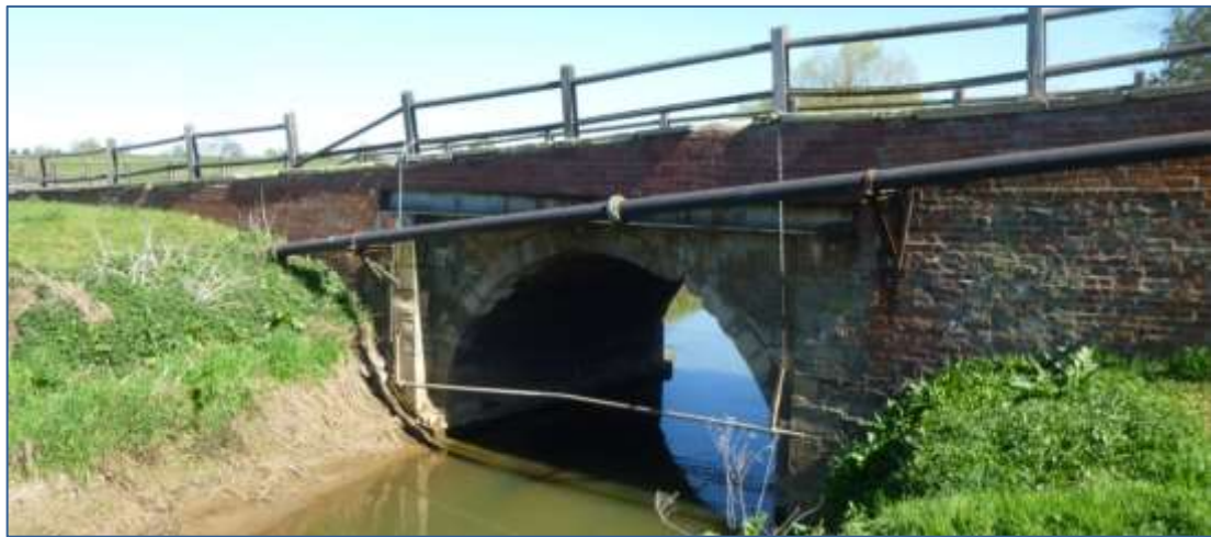
Plate 26: Hagg Bridge, northern span over The Beck.
