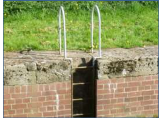
Plates 34-35: Evidence for bumper pieces in Top Lock (left) and modern ladder in East Cottingwith Lock.
